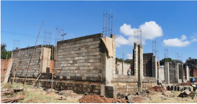
Figure 17: Construction in Progress
